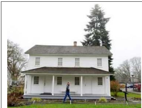
The Methodist Parsonage at the Willamette Heritage Center at The Mill will close after Saturday, Jan. 12, for major renovations. / DANIELLE PETERSON / Statesman Journal
