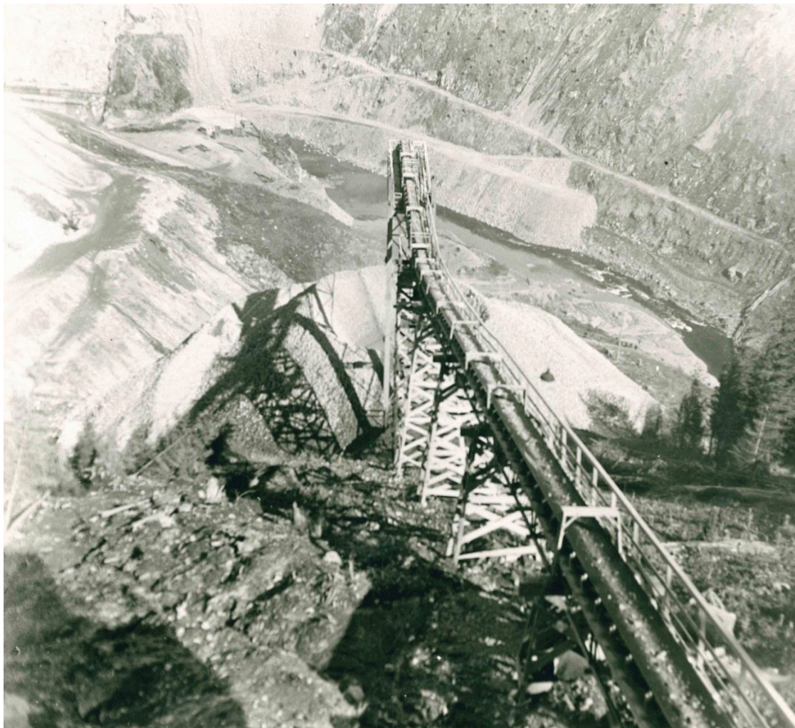
Figure 8. Aggregate conveyer on the south side of the Detroit Dam site. Photo from the US Army Corps of Engineers. WHC #1998.24.16.
