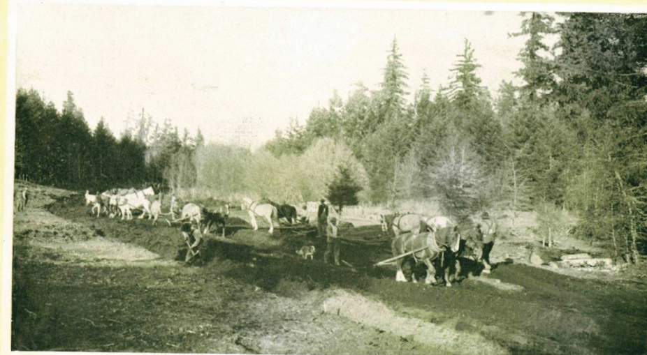
CONSTRUCTING THE WEST STAYTON IRRIGATION CANAL (April, 1911)
