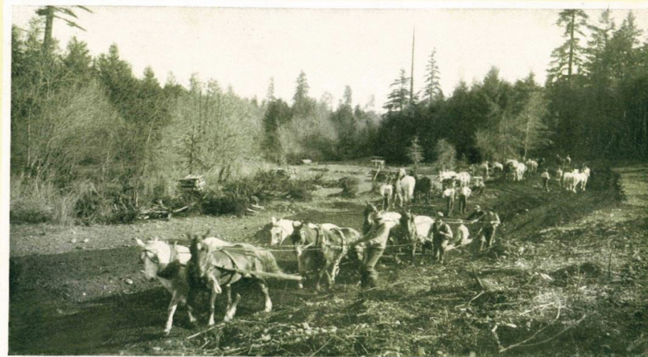
PLOWING THROUGH A BIT OF TIMBER TO CONSTRUCT CANAL
