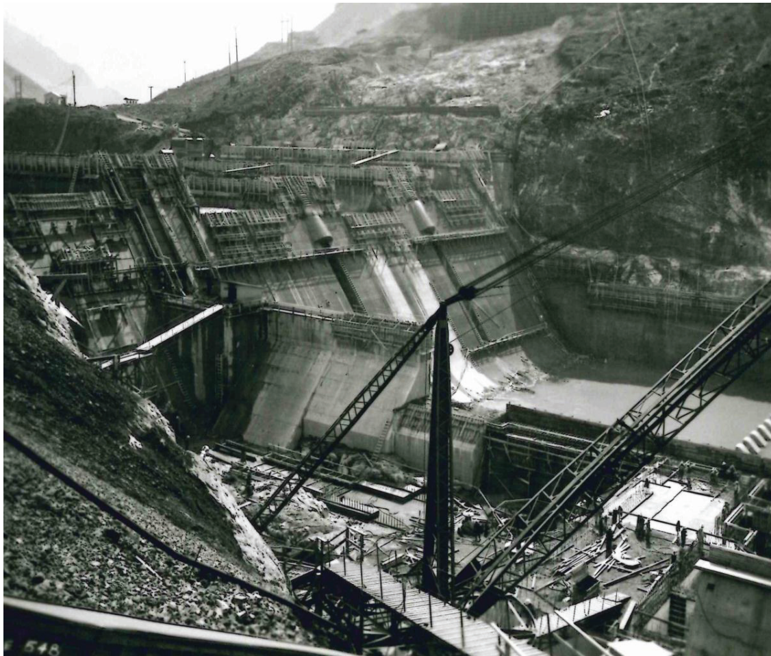
Figure 10. Looking upstream at Detroit Dam showing rebar and the powerhouse in the lower left. Photo by the US Army Corps of Engineers. WHC #1998.25.37.
