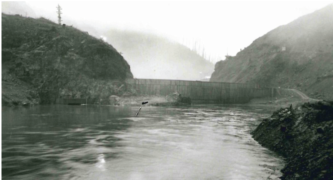
Figure 6. Cofferdam at the upstream side of the Santiam River. Photo from the US Army Corps of Engineers. WHC #1998.25.25.
