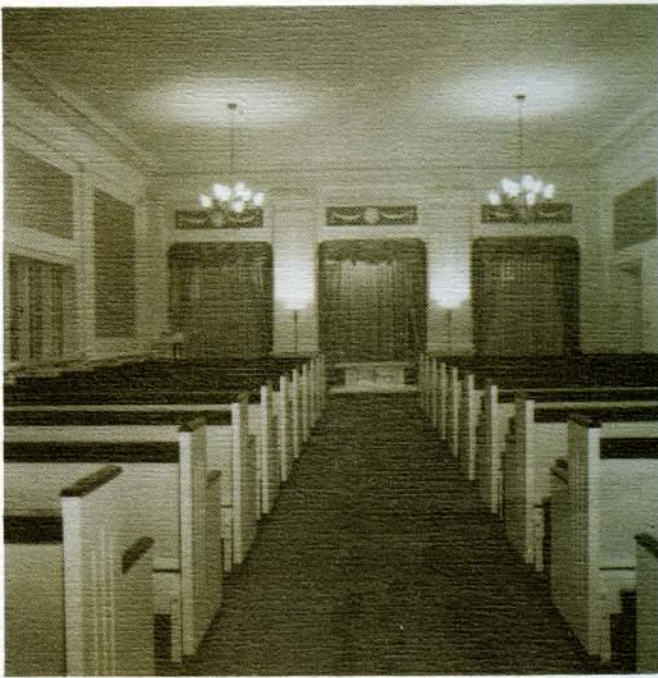
VIEW OF FRONT OF CHAPEL
