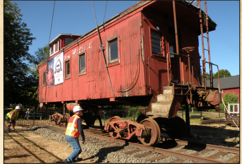
Caboose #507 being lowered onto its new tracks in July.
